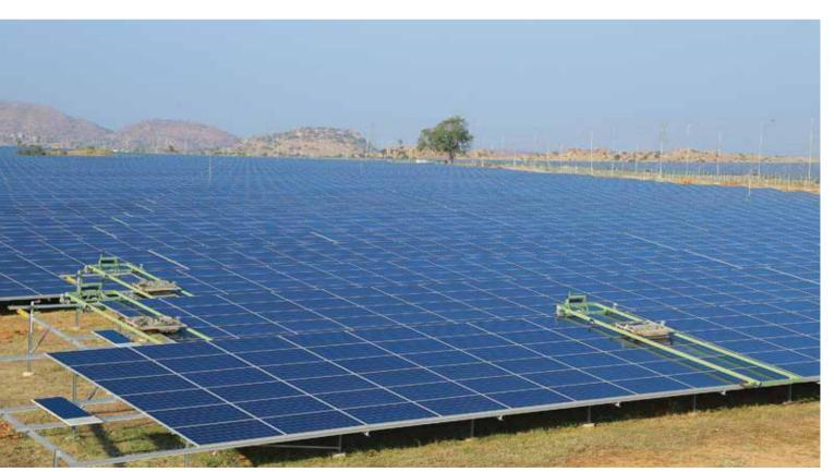
Solar Panel with Robot Cleaning Technology at 2000 MW Pavagada Solar Park, District Tumkur, Karnataka
