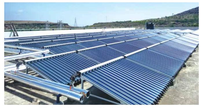
CPC based pressurized hot water system installed at Asian Paints Ltd., Khandala, Maharashtra
